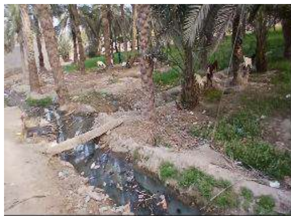
Inadequate drainage of wastewater is contributing to risks for surrounding biodiversity
