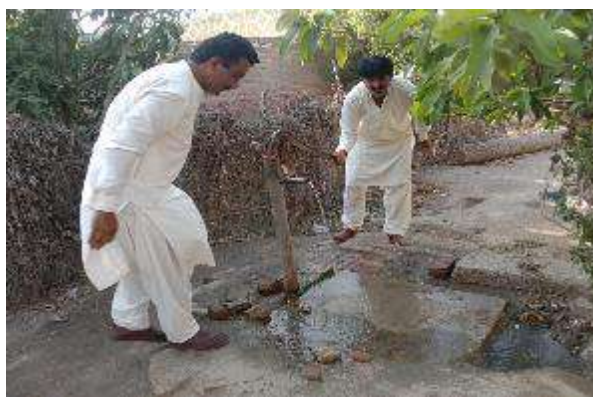
The communal handpumps, existing source of water supply
