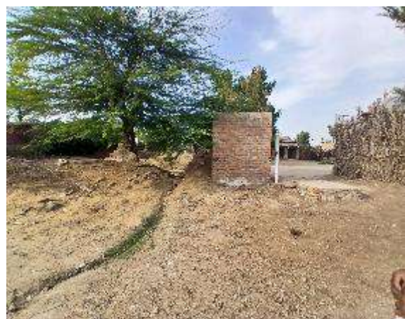
Non-engineered washroom in village
